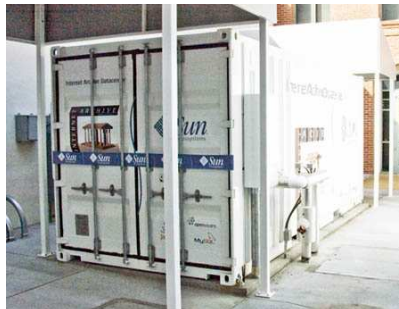
Figure 7.41: This shipping container holds the entire Internet Archive. Potentially, portable data centers could be moved to places which had unexpected need for intensive data storage and processing. (check permission)
