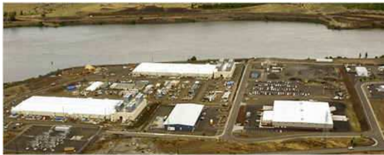
Figure 7.40: The Google data center in The Dalles, Oregon. Dams on the Columbia River (background) provide hydro power. (check permission)
