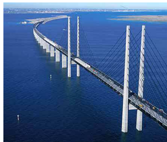
Figure 8.60: Large scale project management is needed in complex projects such as the construction of the Oresund bridge [?].
